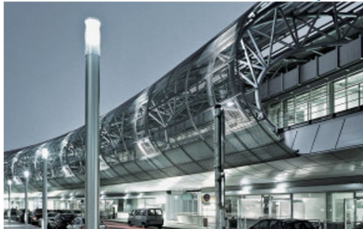
Solar-shades at the Dusseldorf Airport
